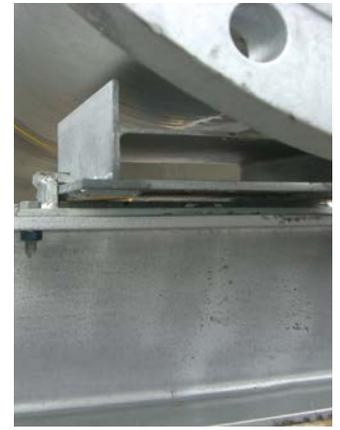
The custom Anvil Fig. 439 Structural "H" Slide Assembly is in place to support the deluge system pipe.
