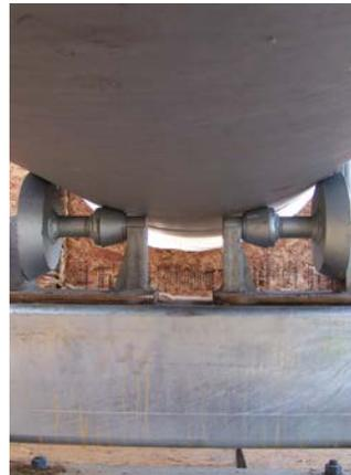
Customized specifically for the unique application, the Anvil Fig. 76SD Fabricated Roller.
