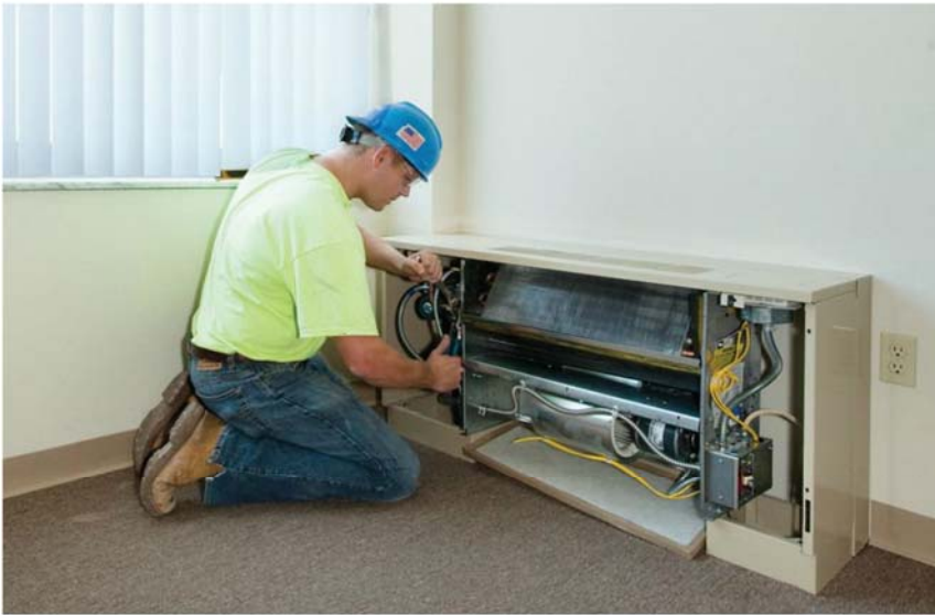
Left: The Taco LoadMatch pumps are shown inside one of the fan coil units in an apartment at Council Tower. The building contains 402 console-type Airtherm fan coils. Right: The use of vertical in-line pumps requires less start-up time since field alignment of the pumps is not required.
