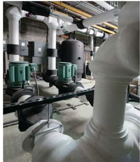
Left: The Taco LoadMatch pumps are shown inside one of the fan coil units in an apartment at Council Tower. The building contains 402 console-type Airtherm fan coils. Right: The use of vertical in-line pumps requires less start-up time since field alignment of the pumps is not required.
