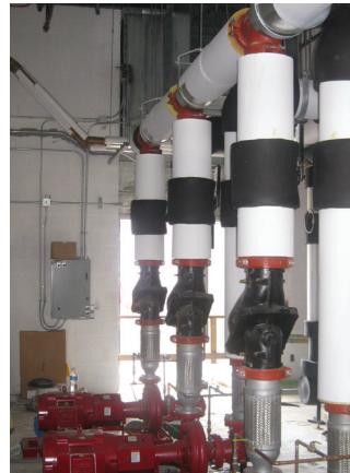
A series of Gruvlok components from tri-service valves, couplings and braided flex connectors.
