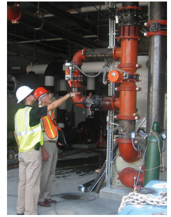
Demonstration on ease of installation when Gruvlok products are used.
