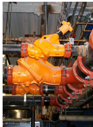
Gruvlok balancing valves and AnvilFlex™ flex connectors (left photo) and Anvil tri-service and butterfly valves (right photo) provide a high-quality piping solution for the new community center.
