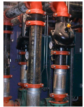
Gruvlok balancing valves and AnvilFlex™ flex connectors (left photo) and Anvil tri-service and butterfly valves (right photo) provide a high-quality piping solution for the new community center.
