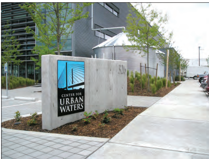
Eagle Harbor Mechanical installed a rainwater harvesting system in Tacoma, WA's Center for Urban Waters building, relying on Jay R. Smith Mfg. Co.® products to do the job. The visible stainless steel water storage tanks draw attention to rainwater harvesting and the city's efforts to promote sustainability.
