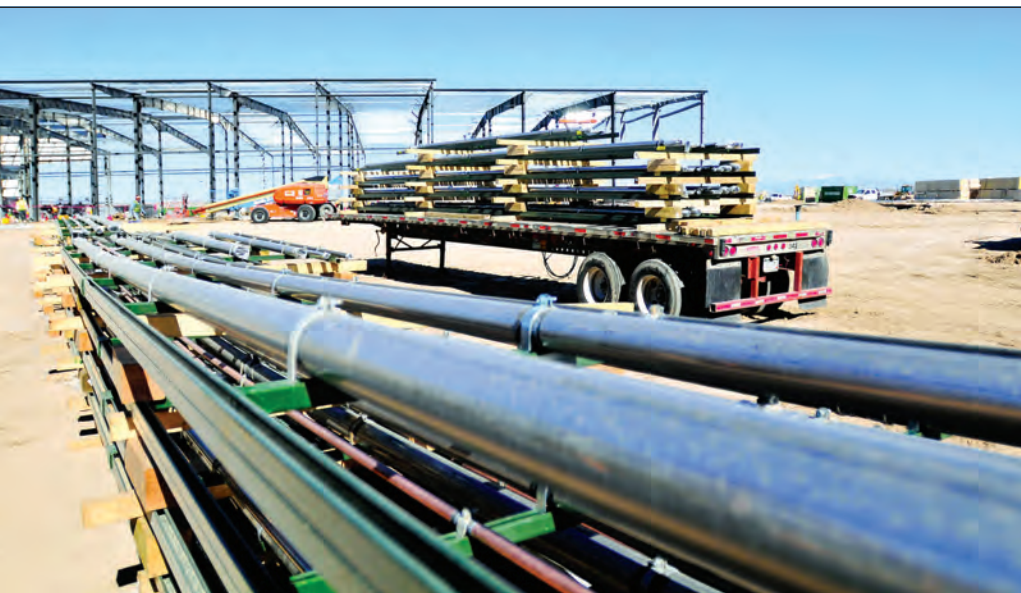
"The prefabricated piping lines had to be trucked to the Pueblo facility from the Olson Plumbing and Heating headquarters in Colorado Springs ... on 40-foot racks," said John Hill, superintendent of Olson Plumbing and Heating. "We worked in two teams of three and installed 21 miles of stainless pipe."
