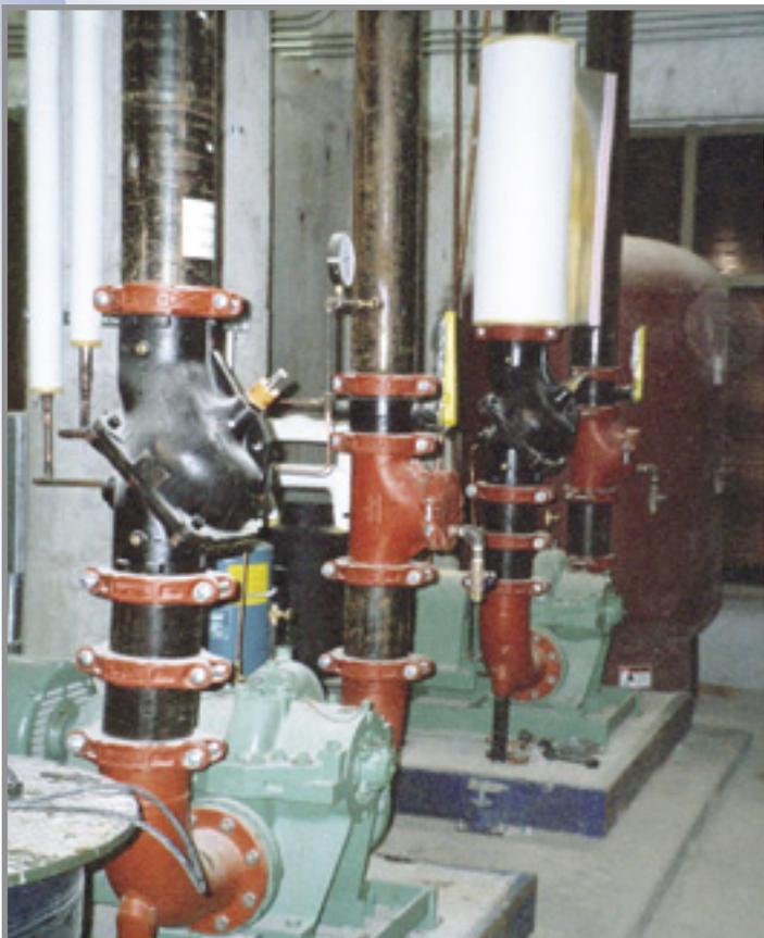
**Flex Couplings keep Pump Components at Serviceable Height**
