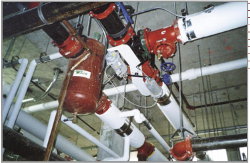
**Easy Access 3-Way Valve, Tee Strainers, and Air Separator (Located Together)**
